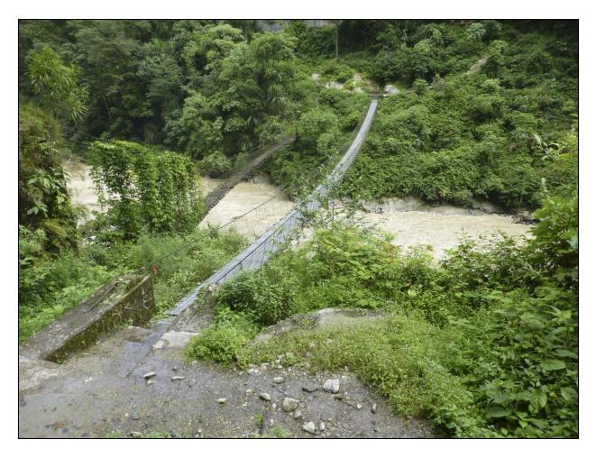
**Figure 4.** The metal cable bridge today. The old wooden bridge which replaced the bamboo and rope bridge of the 1970s can be seen to the left, or downstream, of the new metal cable bridge (photograph by A. Byers).
