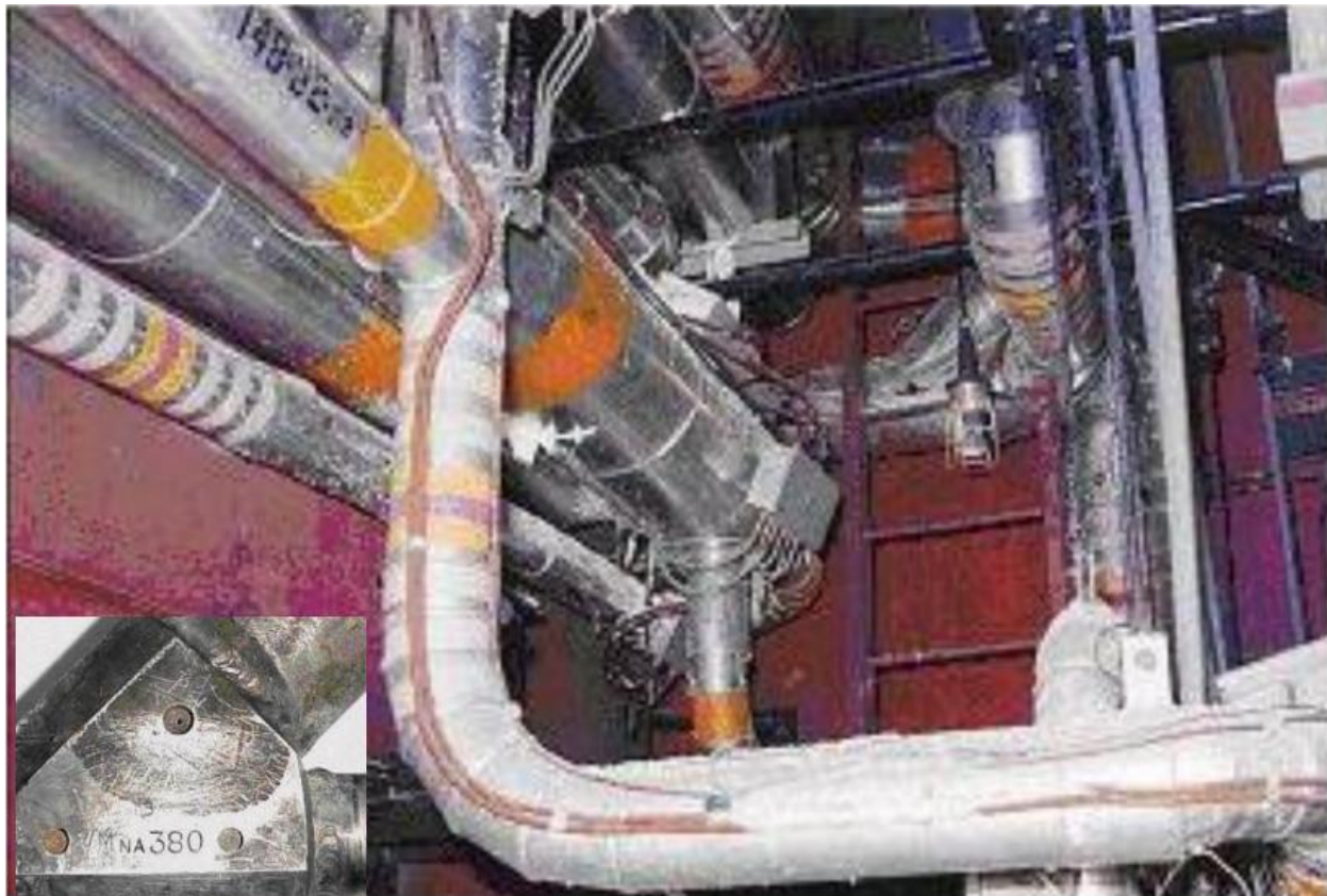
Figure 128. Sodium leak location on FBTR [104].
